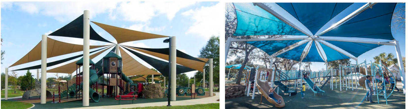
Figure 5.16 - Structures d'ombrage centrales
